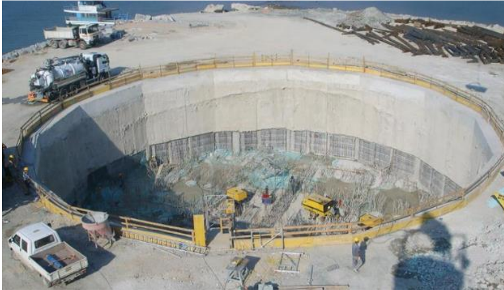
Picture 6 Foundations of the pylon
