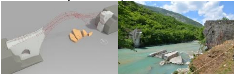
Figure 8: Bridge Collapse (01 Feb. 2015)
