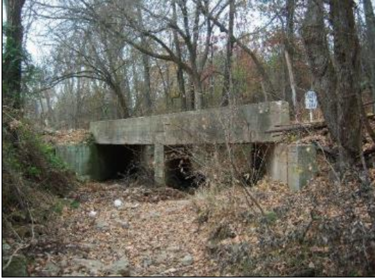
Figure 2: 2014 photograph of culvert north of Ritchey (Courtesy: Harold Dale Barlow)
