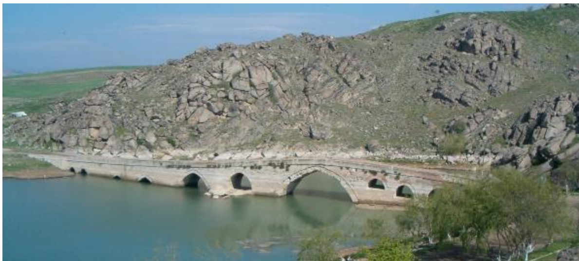
Figure 1 Ceşnigir Bridge over Halys River (Photo: Kantaratlas-2010)
