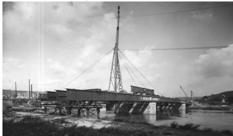
Fig 8: New Herdecke Bridge under construction Germany, 1951 Source: BMVI
