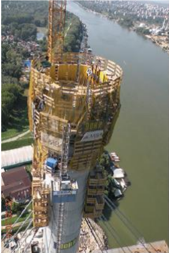
Picture 4 Pylon during construction
