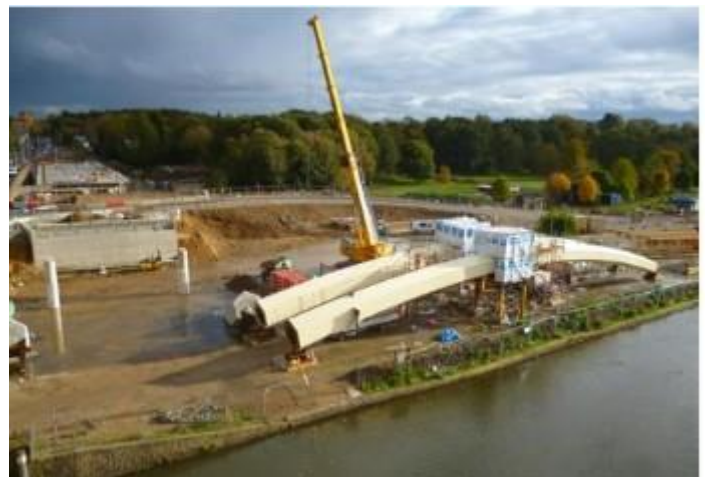
Figure 16: Arch sections being welded together on the river bank ( Costain archives )
