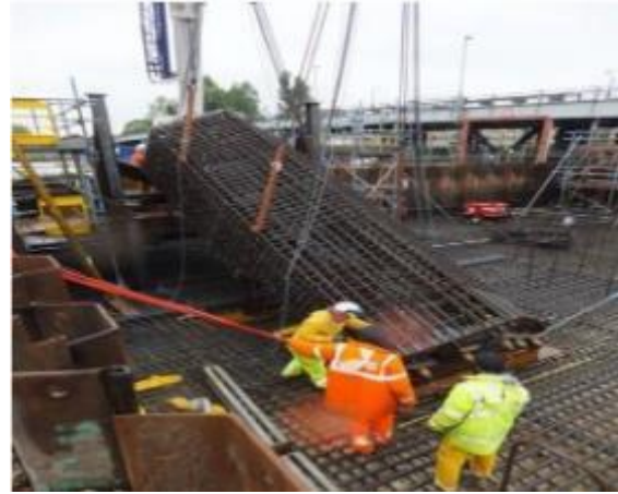
Figure 14: Arch support installation ( Costain archives )
