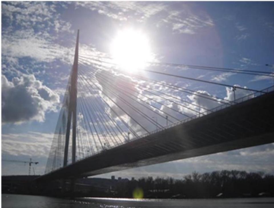
Picture 13 Completed main span and the pylon
