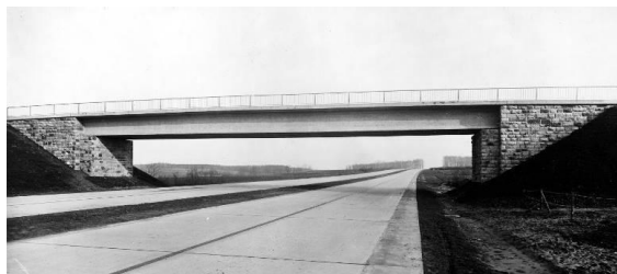
Fig 5: Bridge „Farmer Hesseler“ at Oelde Germany, 1938 Source: HWA Darmstadt
