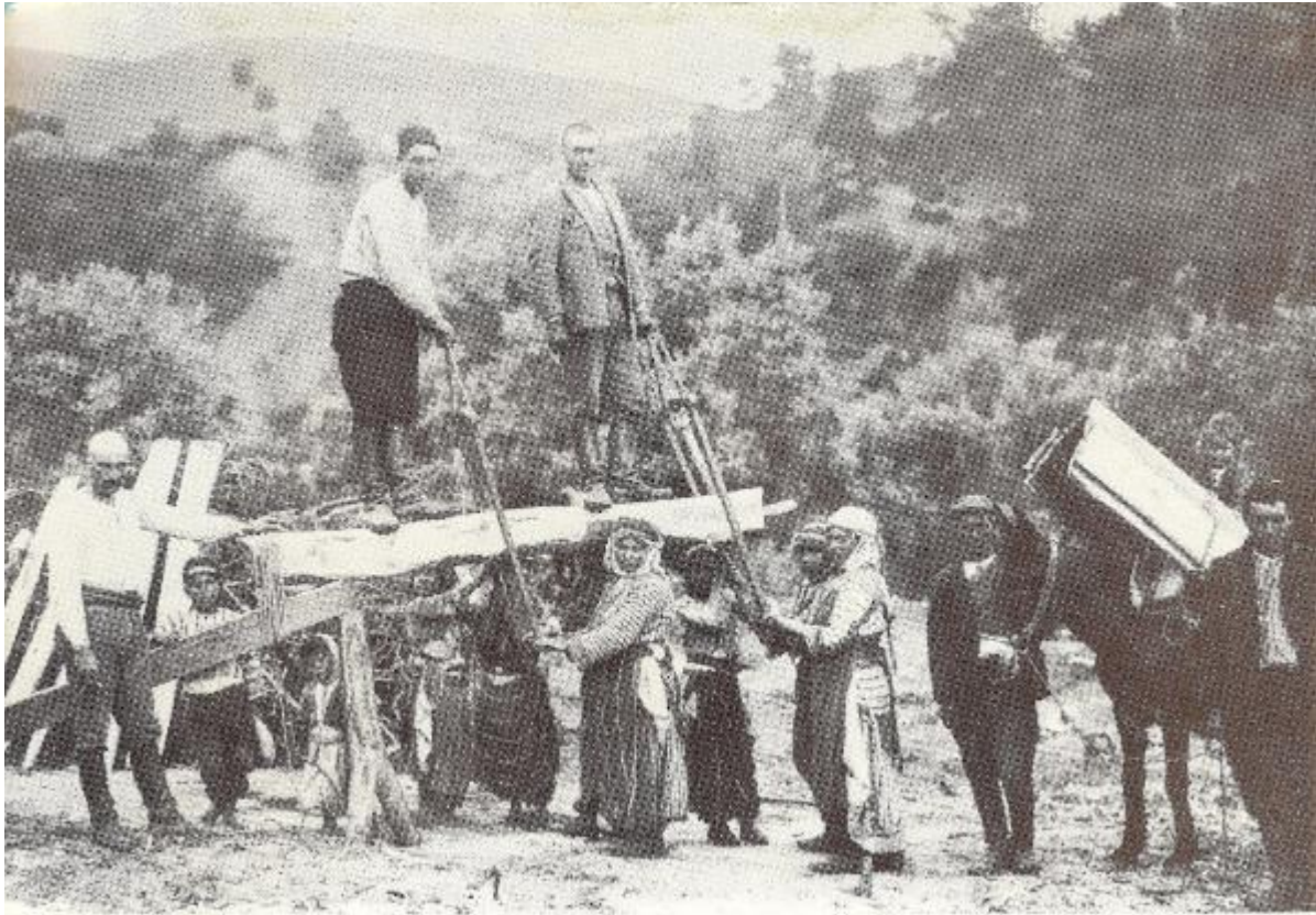
Figure 8 Timber preparation for a Bridge near İzmir (Smyrna) Year 1937 (KGM 1970)
