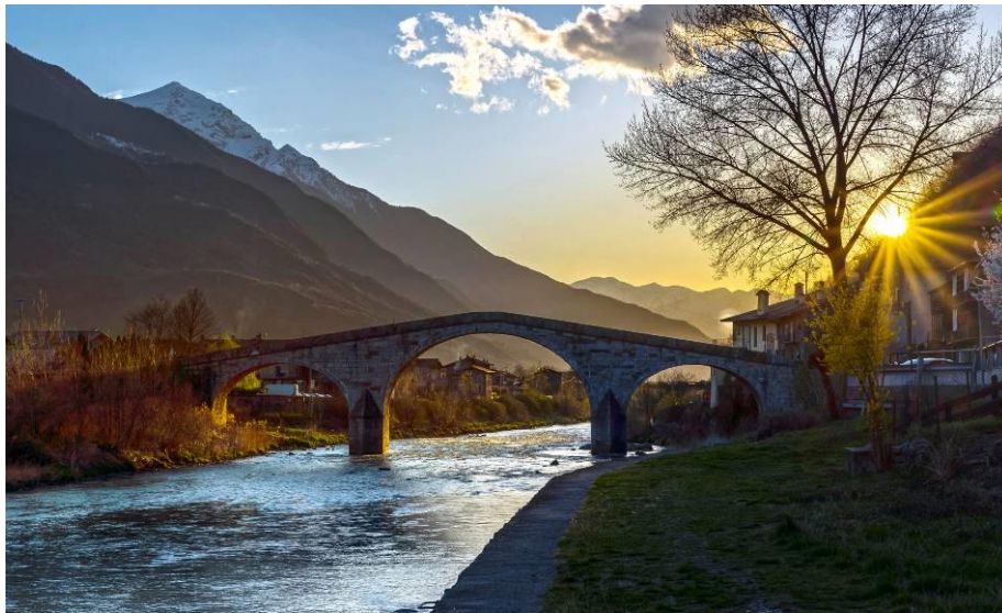
Fig. 1 Ganda bridge in its natural setting
