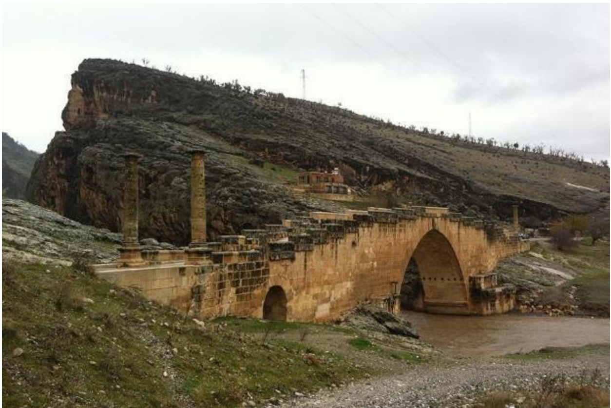
Figure 2 Cendere Bridge over Chabinas River (Photo: İvestadiyaman 2017)
