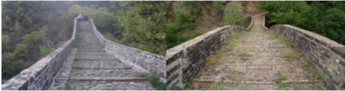
Figure 14: Bridge deck: Recently restored parts (left), original deck (right).
