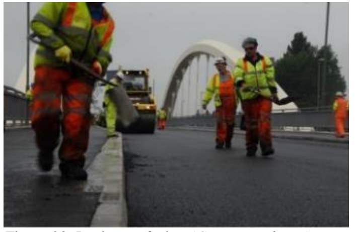
Figure 20: Laying surfacing ( Costain archives )
