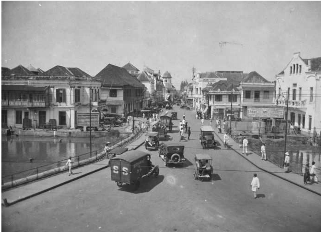
Jembatan Merah, 1920s, entry to the main commercial district. (Source: http://kotawisataindonesia.com/melihat-sejarah-jembatan-merah-di-surabaya/jembatan-merah-surabaya-tempo-dulu/ )
