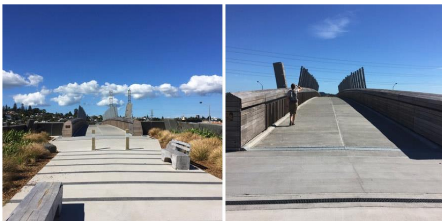
Figure 5a: Taumanu Reserve Bridge, approach from Eastern side. (Photography J. Naismith)
