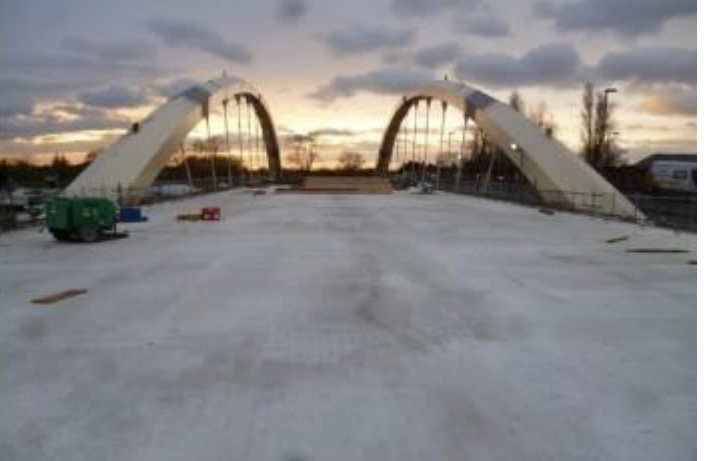
Figure 19: Completion of the concrete deck ( Costain archives )
