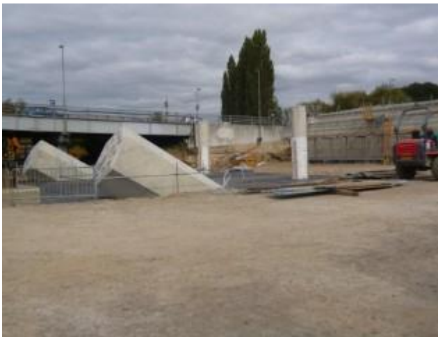
Figure 15: Completed support structures ( Costain archives )
