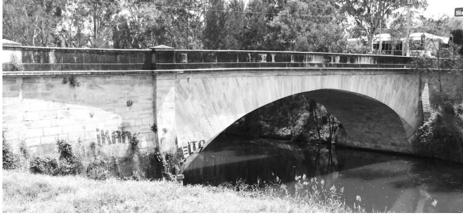
Fig.6 Lansdowne Bridge in 2013.
