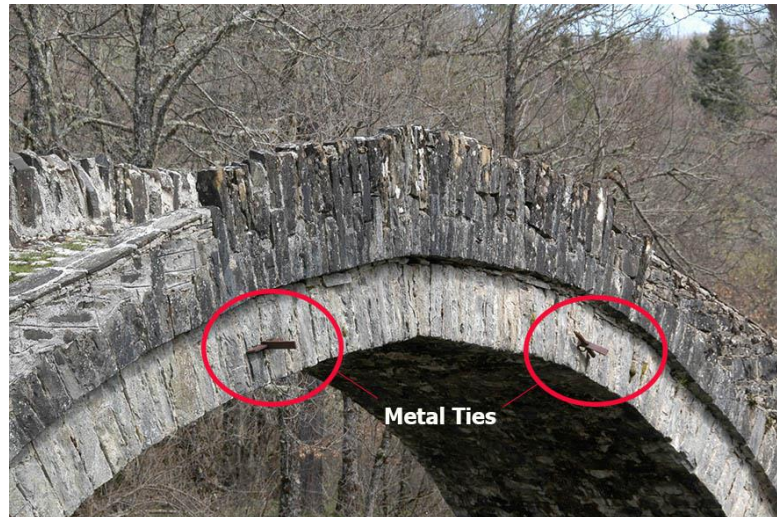
Figure 13.: Detail of metal ties
