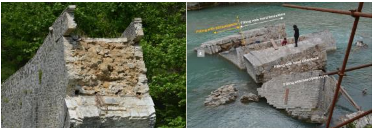
Figure 10: West pier (left). The construction of the outer shell and the inner part of the pier can be clearly seen (the filling with porous stone, the holes of the timber reinforcements in the filling and the construction of the arches). Fallen fragments of the East pier (right). The change of the filling material from limestone to porous stone (yellow line) was occurring at a specific point which coincided with a vertical recess constructed at the outer shell of the bridge.
