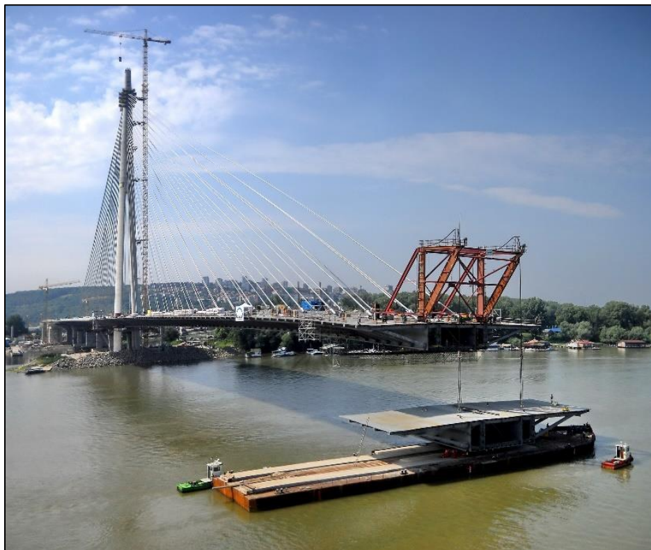
Picture 7 Erection of the steel deck segment
