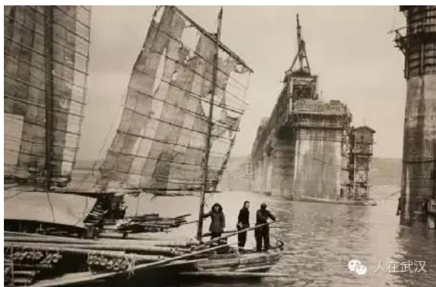
Fig 21. Before the Bridge
