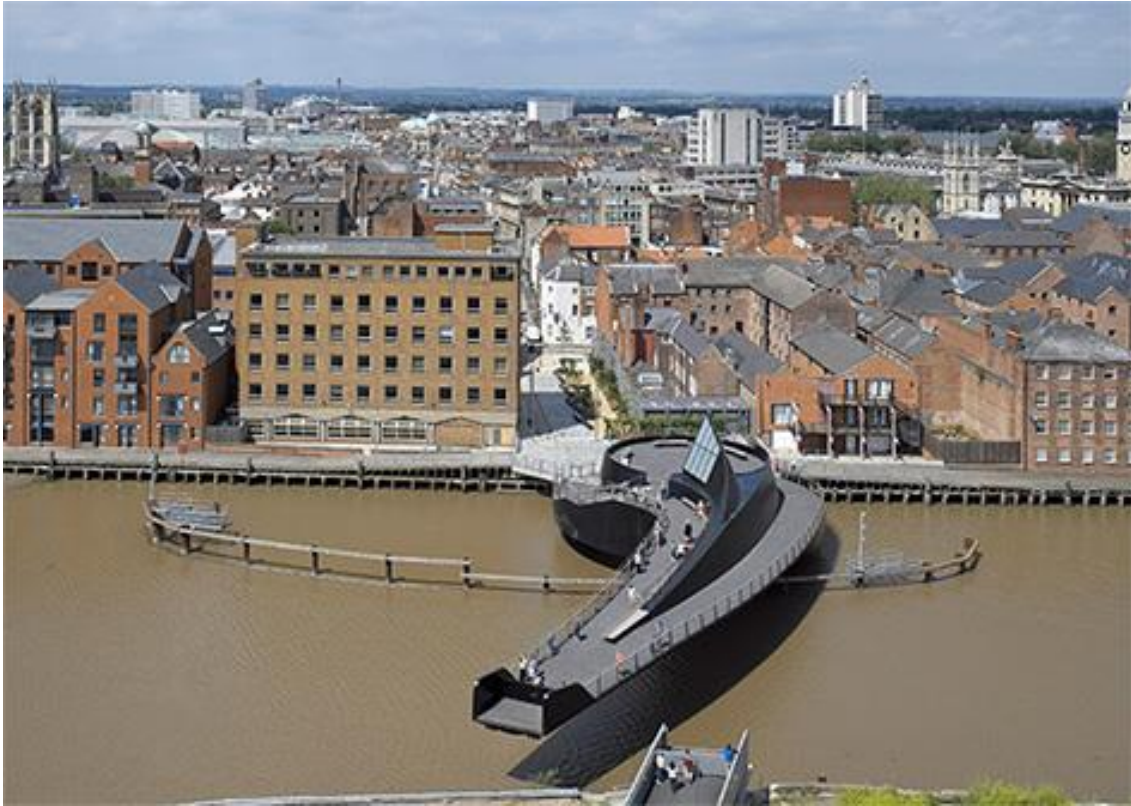
Scale Lane Bridge (photo copyright Tim Soar)
