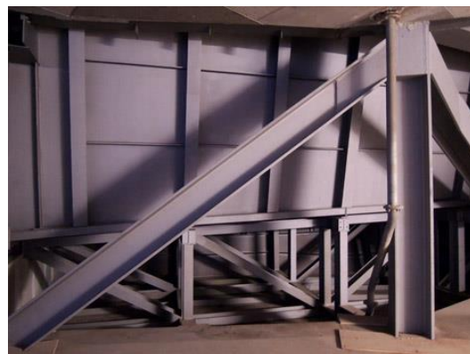
Inside hub space (copyright Matter Architecture)
