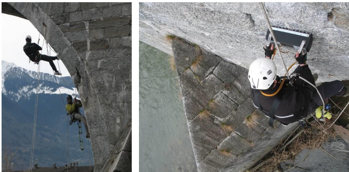
Fig. 7 inspection and ultrasonic measurements performed with positioning techniques by ropes
