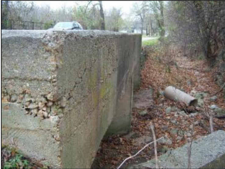
Figure 3: Detail of culvert concrete (Courtesy: Harold Dale Barlow)
