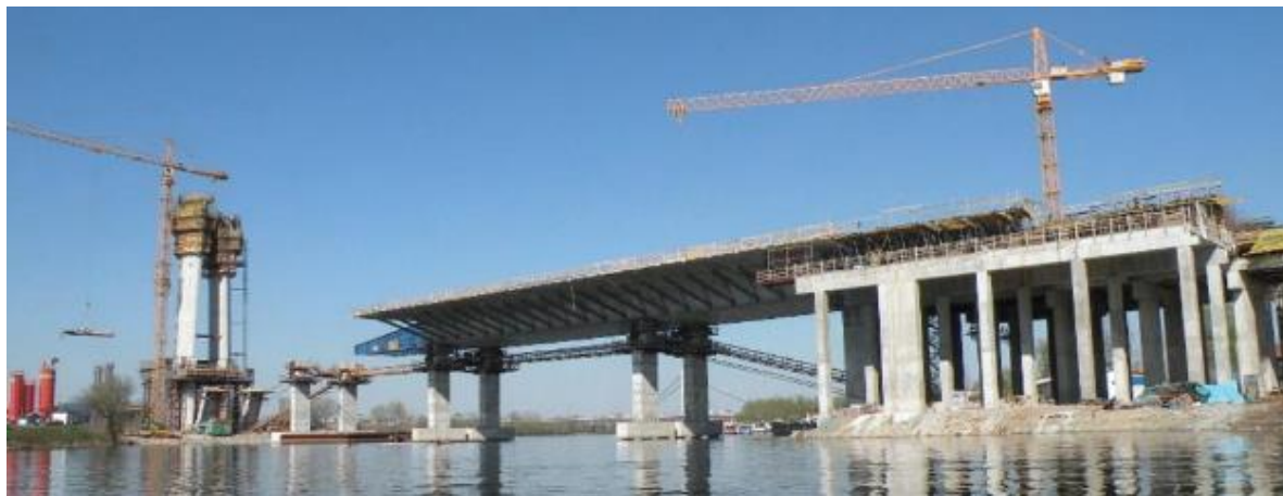
Picture 8 Launching yard and the back span of the bridge
