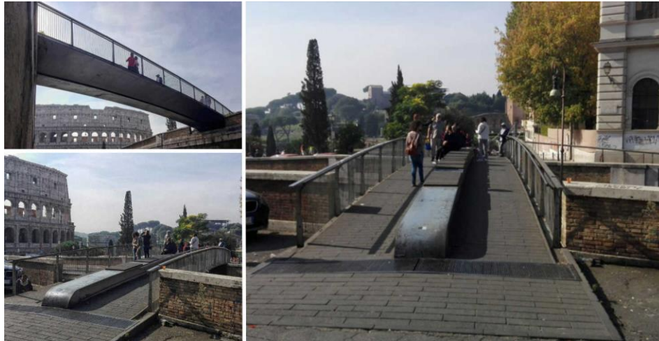
Fig. 7 The Annibaldi footbridge, by Francesco Cellini, Insula architects and Fabio Brancaleoni, Rome, 1999 (photos by Remo Di Felice)
