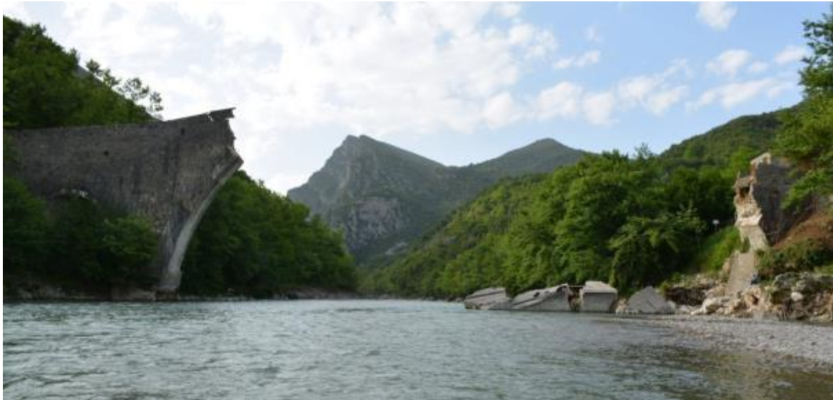
Figure 2: Plaka bridge after the collapse.
