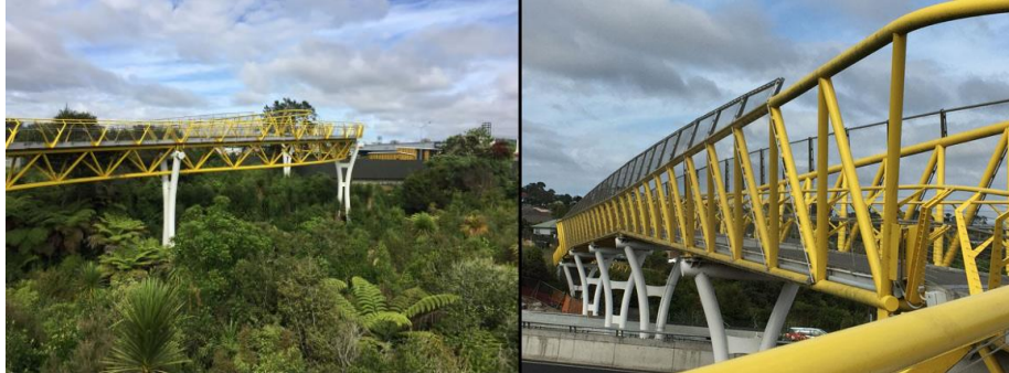
Figure 6a: Westgate Footbridge approach from Mangatewhau Reserve. (Photography J. Naismith)
