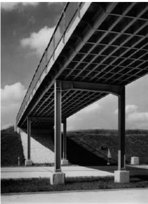
Fig 3: Cellular steel deck Flyover near Juningen Germany, 1936 Source: SAAI Karlsruhe
