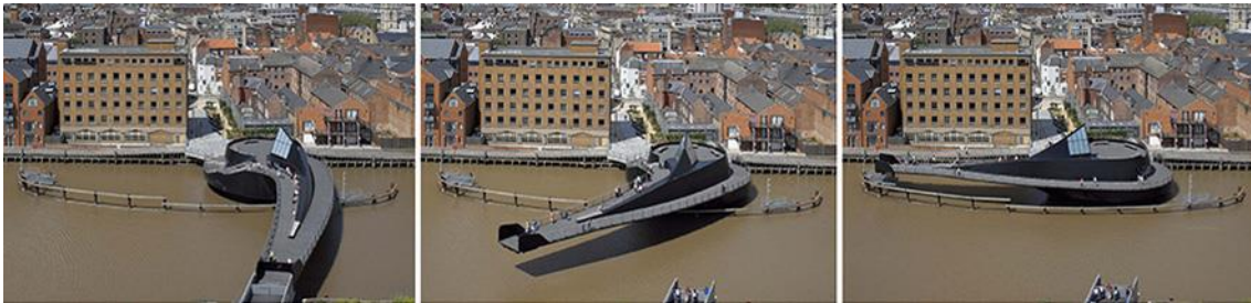
Scale Lane Bridge opening sequence (photos copyright Tim Soar)
