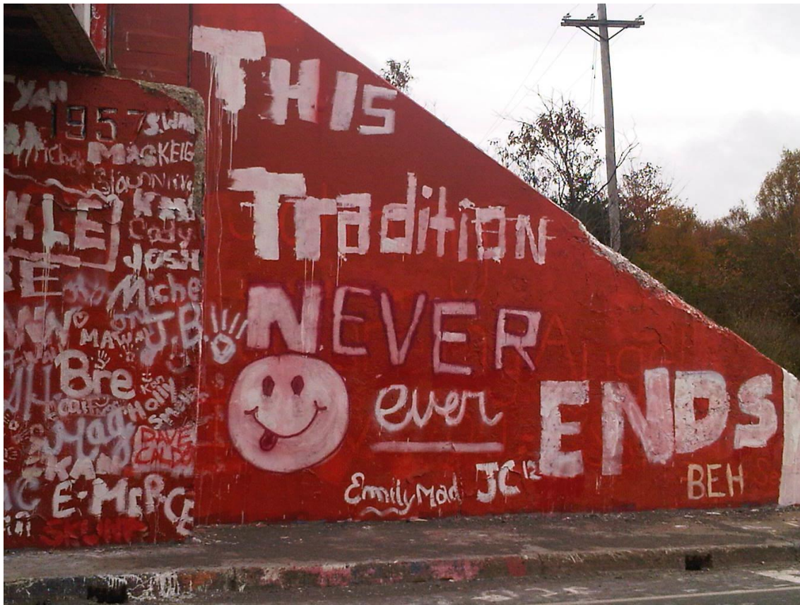
Figure 2. Sydney River Trestle Bridge (Southwest retaining wall), 21 Oct., 2010. Photo by Ian Brodie.
