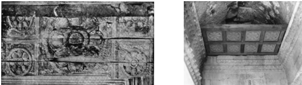
Figure 4: Left- Identification of the old wooden ceiling decoration at Angkor Wat galleries as discovered by Commaile and published in BEFEO 1913. Right- Replacement of the wooden ceiling of the Angkor Wat galleries with cement tiles photographed in August 1948. Source: BEFEO 1913, plate XIX; © EFEO Archive, Paris (Falser Vol. 2:110- fig. IX. 66 a and d)
